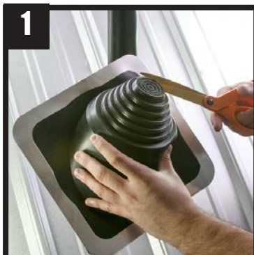
1 Choose pipe opening and trim flashing accordingly.
