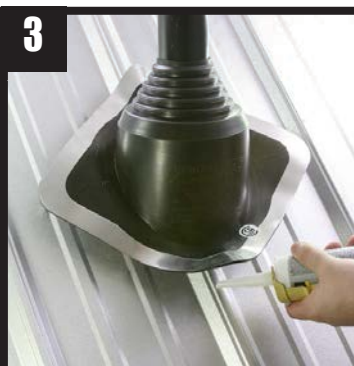
3 Apply sealant to the inside of the flashing about 1/2" in from the outline.
